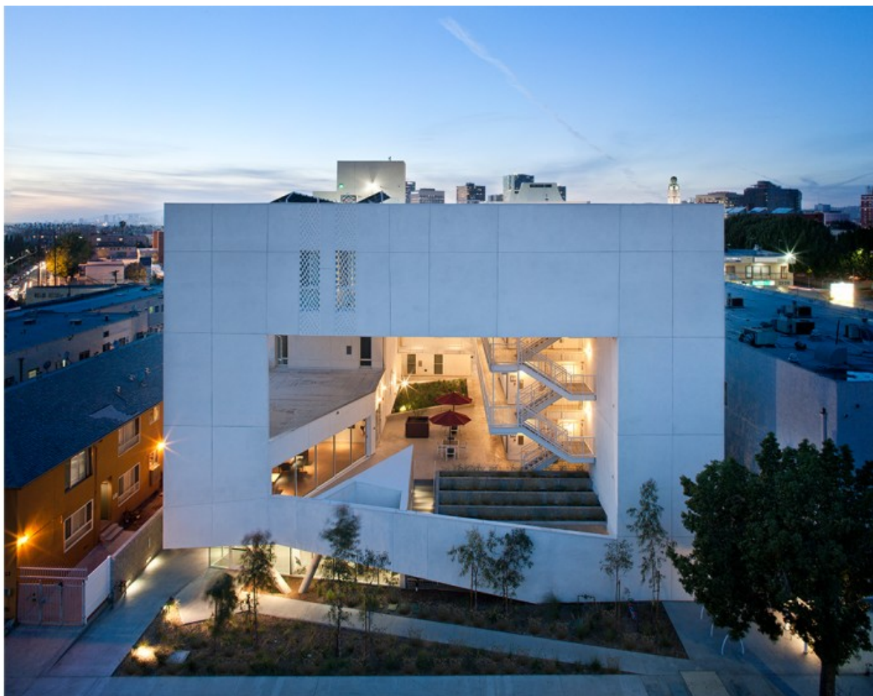
An affordable veterans housing complex called the Six, by L.A. architects Brooks + Scarpa. (Brooks + Scarpa)
